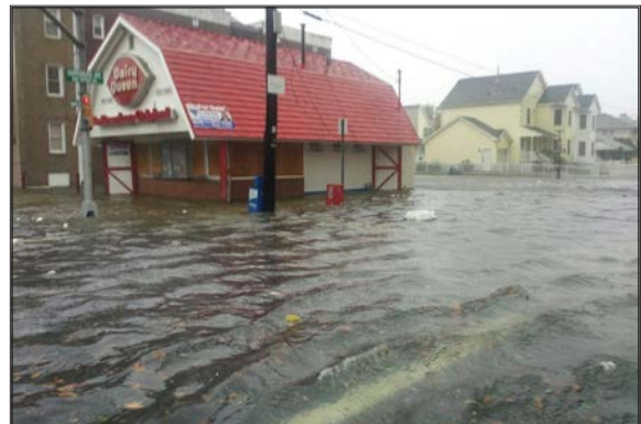
A Dairy Queen in Atlantic City, NJ after Hurricane Sandy struck
