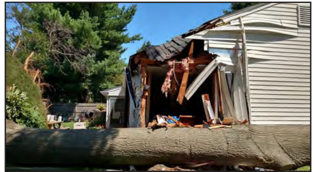
The Yeadons' badly damaged house, with the trunk of a huge uprooted tree in the foreground
